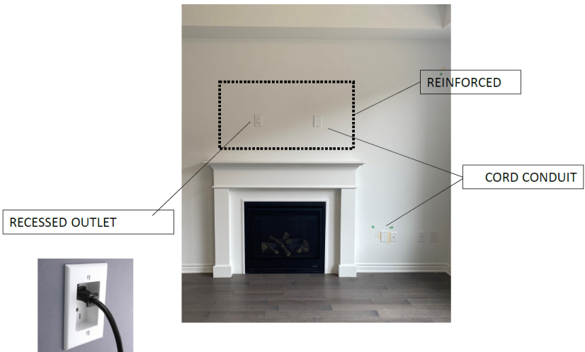
Wall Mounted TV Framing (With Conduit)
