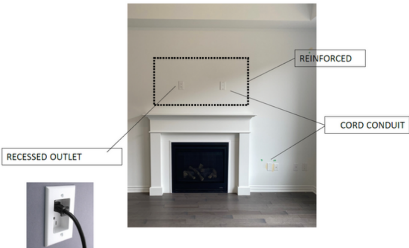
Wall Mounted TV Framing (With Conduit)
