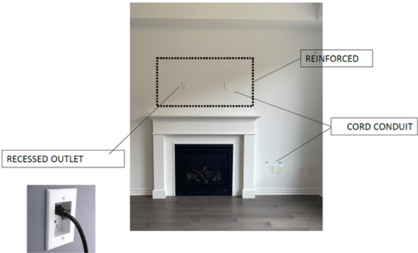
Wall Mounted TV Framing (With Conduit)
