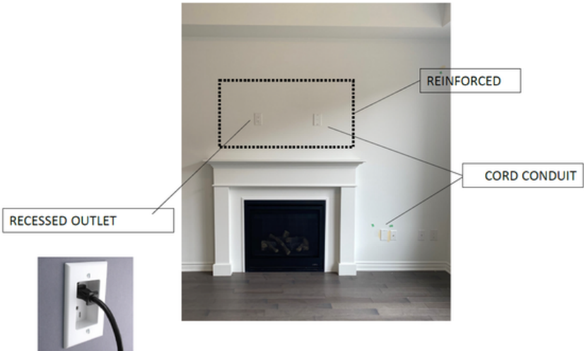
Wall Mounted TV Framing (With Conduit)
